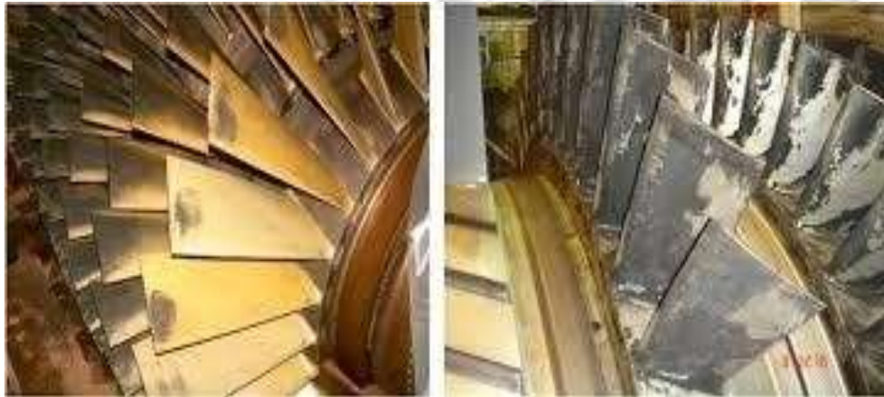
Fig. Compressor blade fouling
